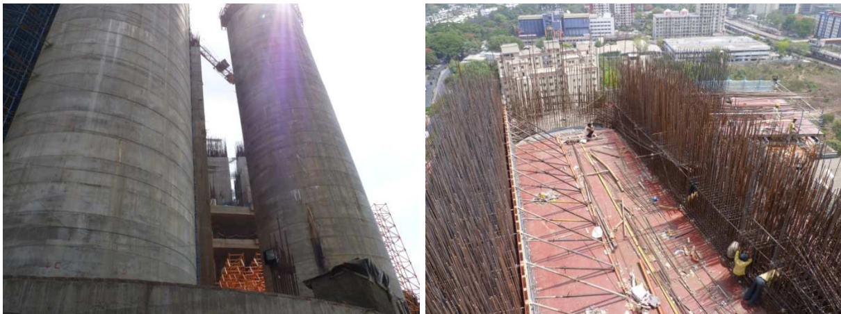
Fig 8: The Columns and the girder beam(Top view) which is being monitored.
